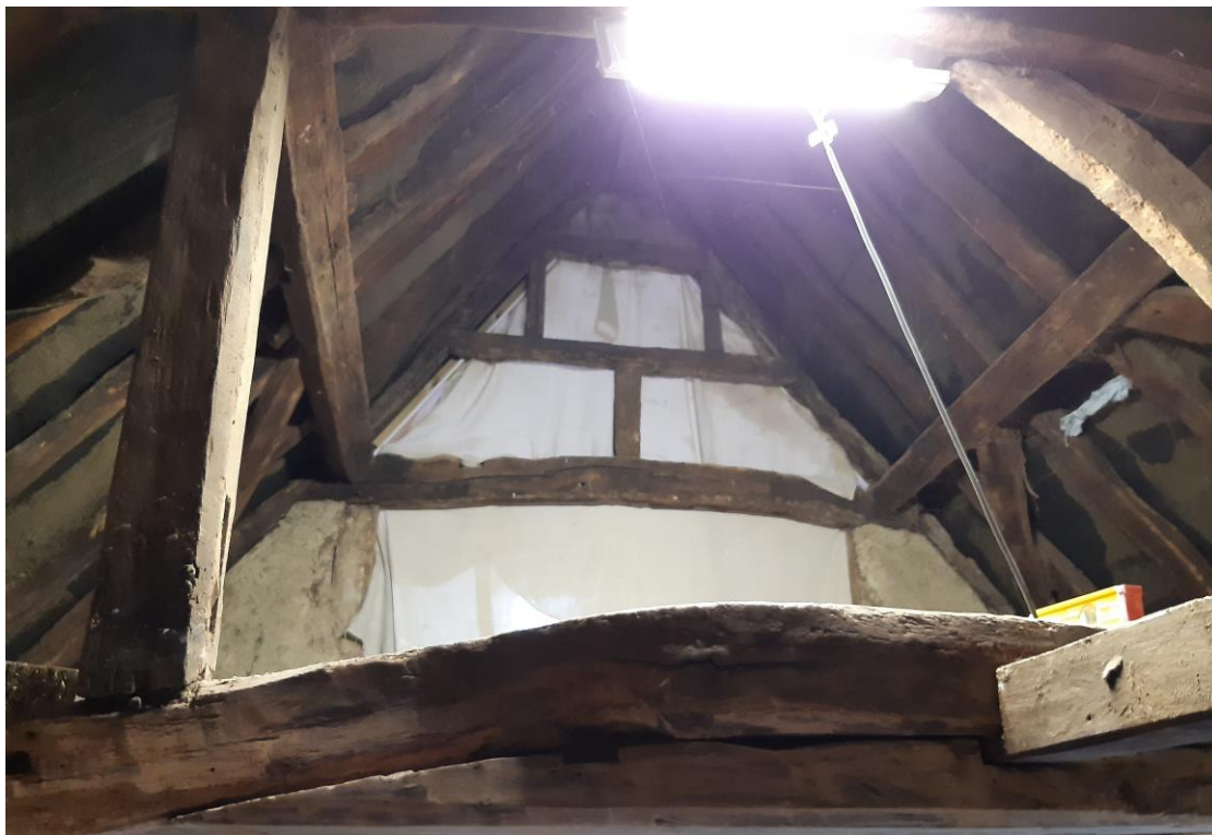
Image – Roof structure, Old Bakehouse, N. Crawley
